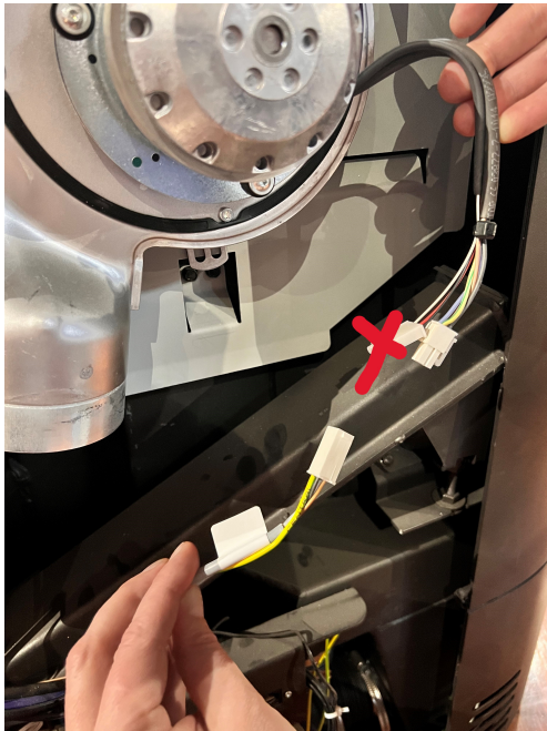
Fig. 20: Connecting the cables
