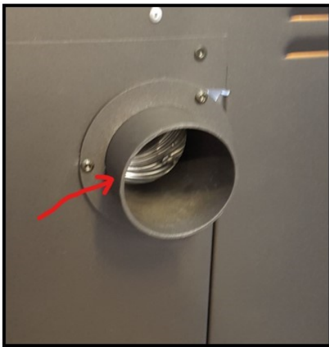
Fig. 14: Installer le raccord double
