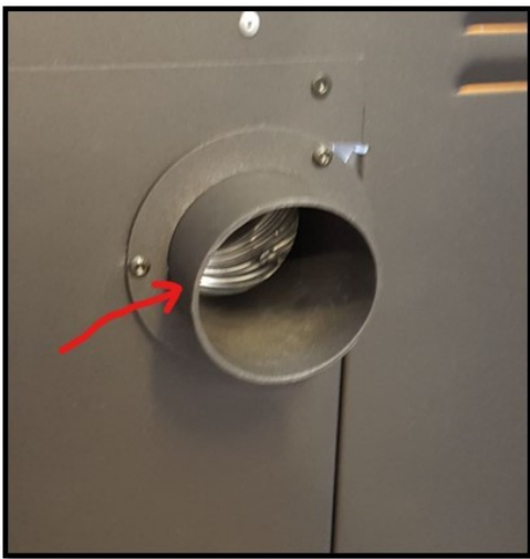
Fig. 72: Installer le raccord double
